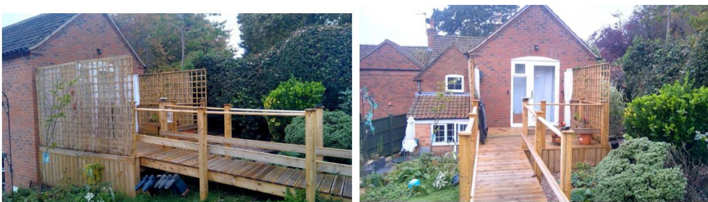
Fig. 5 Site Photos of Development
